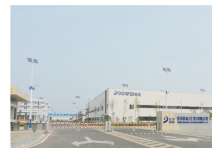
宿迁工厂 Suqian Plant
